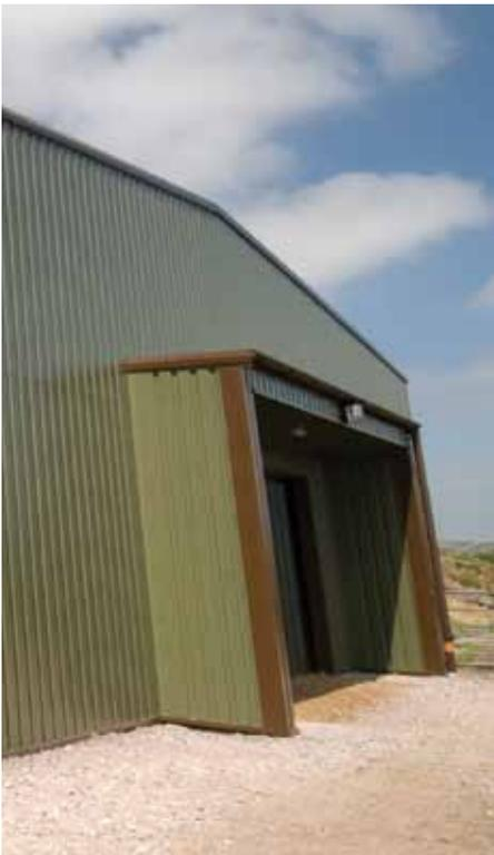
Ruralclad® is a value pre-finished steel product, designed for agricultural buildings that would only be used for dry storage e.g. implement sheds. Produced to the high quality standards expected from Tata Steel, it consists of a galvanised substrate with a nominal 18µm flexible paint system on the exterior side of the sheet and a standard high performance reverse side backing coat.
