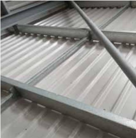
Colorcoat® PE 25 is an economic product suitable for undemanding roof and wall applications particularly in dry and non-aggressive climates where there are no high demands for corrosion protection.
